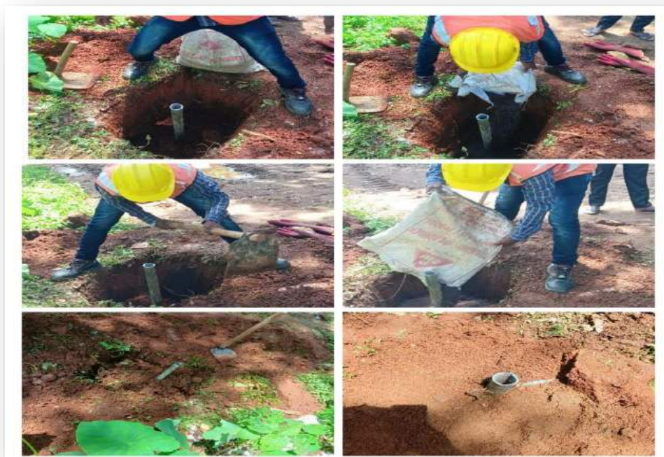
Picture 15: Earthing installation at DSS
