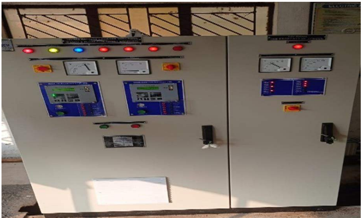
Picture 10 : Battery Charger Installation
