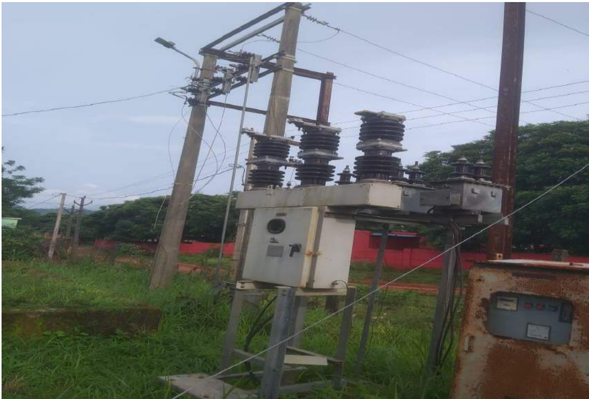
Picture 2 : PSS Refurbishment Required (B)
