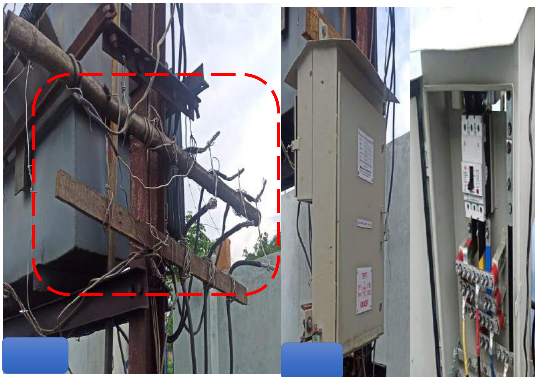
Picture 17: MCCB Installation at LT Protection of DSS
