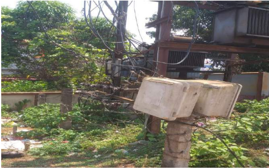
Picture 6 : DSS Refurbishment, DSS LTDB & DSS Fencing Required (B)
