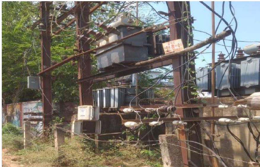
Picture 6 : DSS Refurbishment, DSS LTDB & DSS Fencing Required (B)
