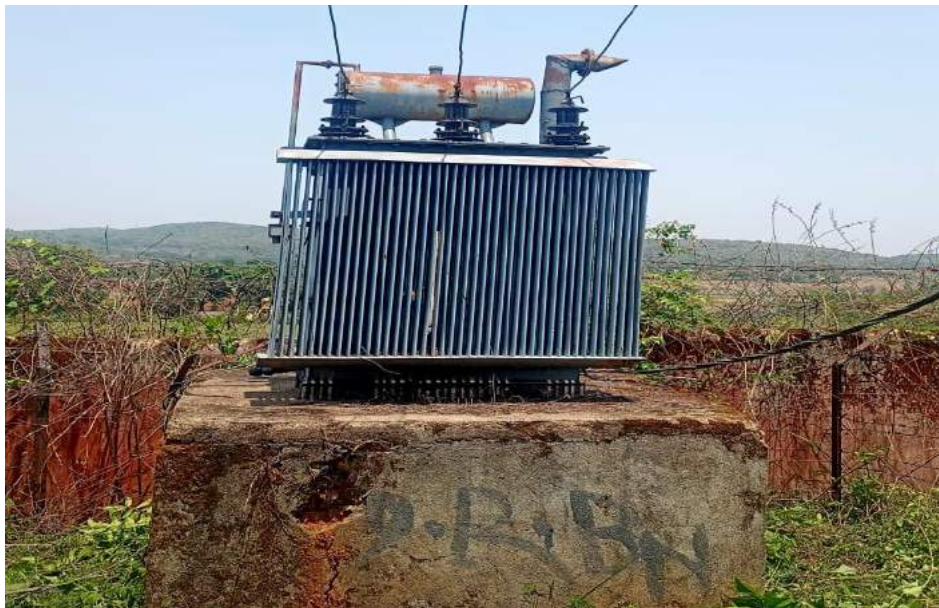
Picture 8 : Building Civil Work, DSS Damage Plinth & New Plinth Work,& PSS Boundry wall Required (B)
